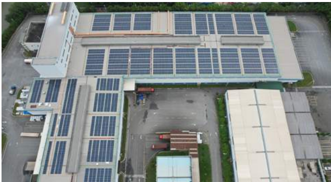
Two major projects to install around 8,000 solar panels were completed at sites in China – helping to accelerate our ambition of cutting carbon emissions in half by 2030. The panels were installed at two of our Decorative Paints plants – more than 5,000 in Shanghai and almost 3,000 in Guangzhou – representing further progress for our greener manufacturing plans.
