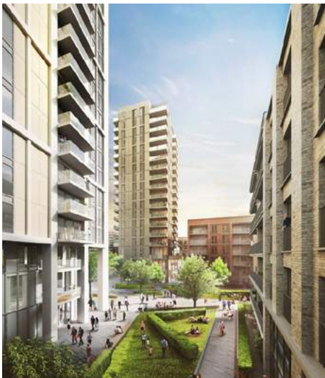
One of London's oldest areas now houses a new residential development which has gone way beyond common methods of reusing and recycling. The buildings of the Silk District in Whitechapel are mainly constructed from brick and reconstituted stone. Our Interpon D Stone Effect powder coatings were applied to the exteriors to imitate the look of Portland stone, limestone and brickwork – helping to preserve the natural materials.
